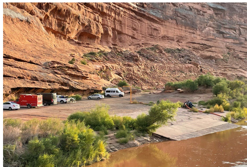
Figure 2: Boat ramp and parking area from pedestrian bridge. Credit: B. Byrne
